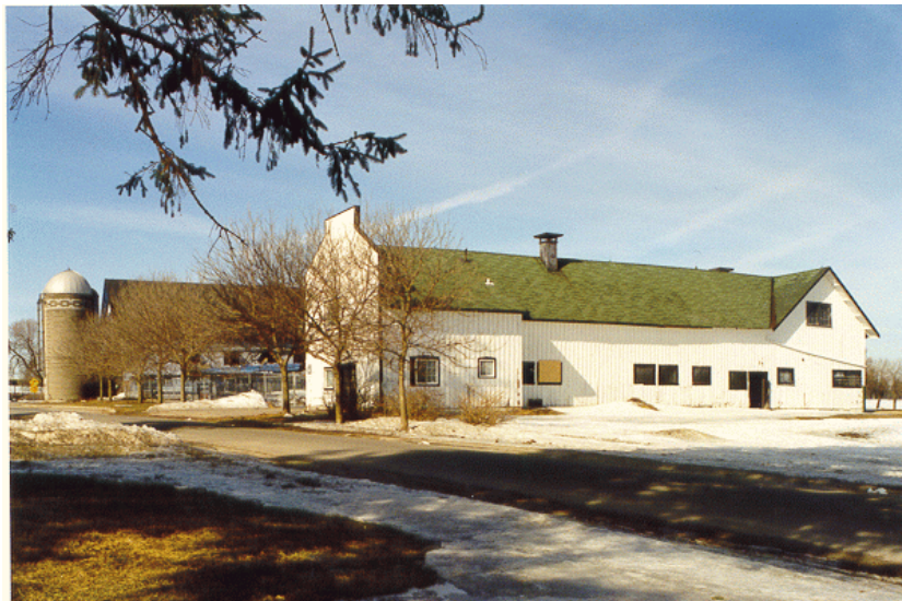
2. Views of Booth Barn Complex, facing north west
