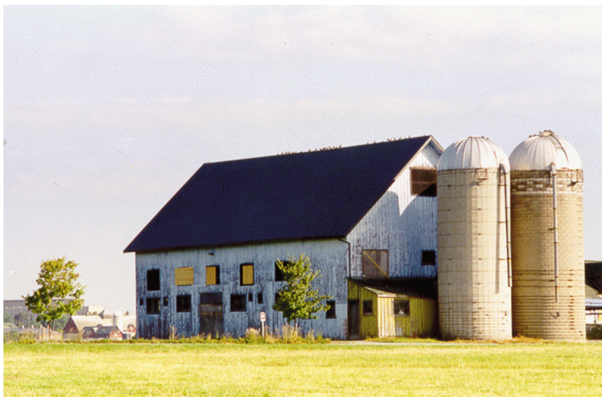
1. Views of Booth Barn Complex, facing north east
