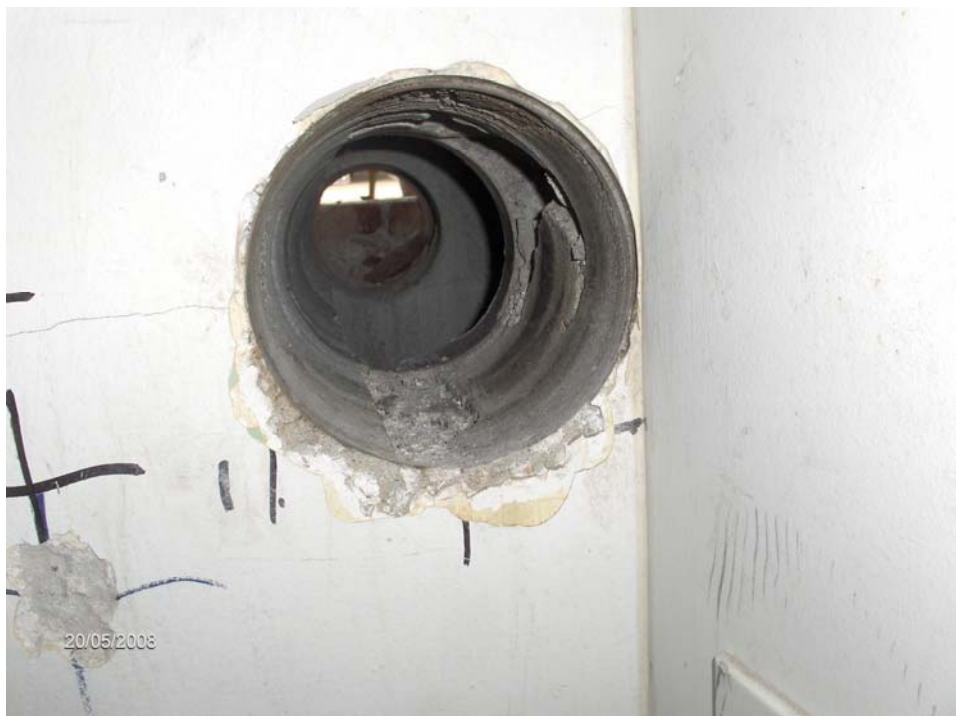
Picture 12 Core sample at the ground floor
