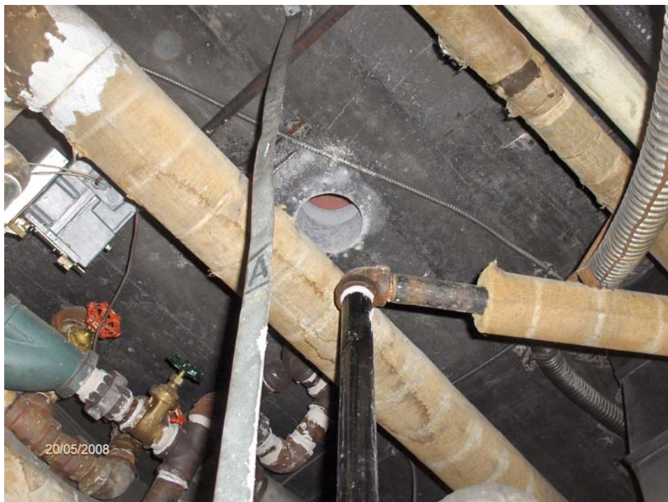
Picture 14 Core sample through ground floor slab
