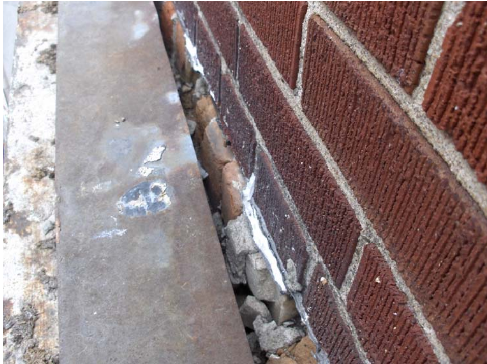
Picture 7 Metal Feature Strip at third floor windows
