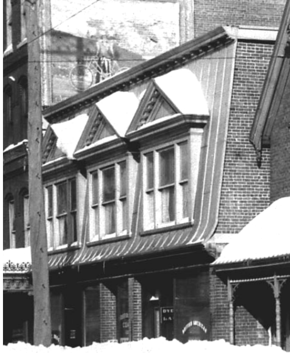
Fig. 1. Historic photo showing lower floor divisions into two larger bays and one small central bay.
