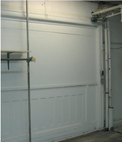
Fig.6 Upper floor, northern portion, showing typical early-twentieth century trim details.
