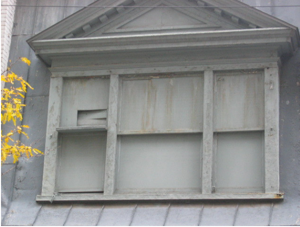
Fig.8 Mansard roof with original standing-seam metal roofing, dormer with dentilled cornice, and original window sash in two of the three frame units.
