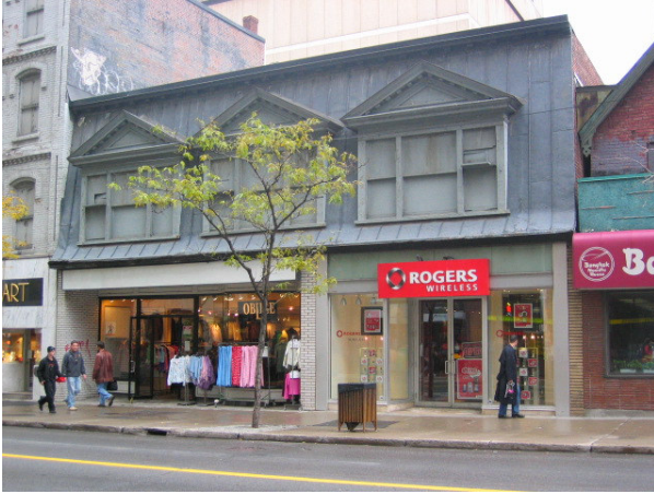
Fig. 3 Current appearance. A single modern storefront on the left replaces the earlier two bays. Also visible in this photograph is the lack of alignment of the southern bay (on the right) with the pattern established by the dormer windows above.
