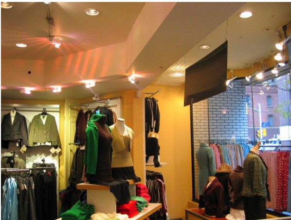
Fig.5 The current retail space on the ground floor of the northern bays. The boxed-in beam contains one of the 14" north-south steel beams. The front façade does not have one of these transverse beams, but is carried by the cantilevered 8" steel beams above.
