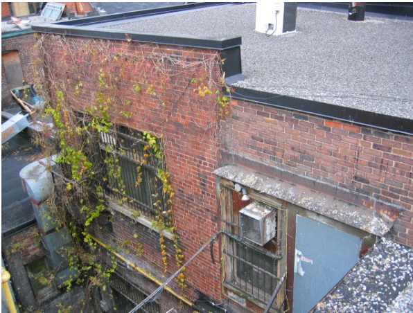
Fig. 2 Rear elevation showing building divisions – south and central bays
