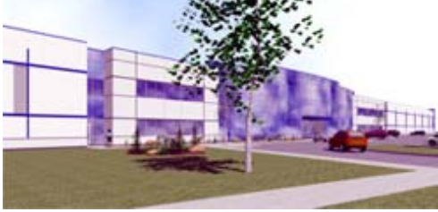
Smart Technologies' new 24,150-m 2 facility on Palladium Drive in Kanata opened in 2007.
