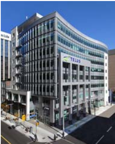
Now open: Telus’ new Ottawa headquarters at Bank and Slater Streets.
