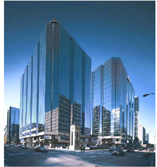
Under construction: Minto's 180 Kent (Minto Place Phase III), a 34,500-m 2 , 19-storey, LEED-Gold certified office tower that will be ready for occupancy in 2009.
