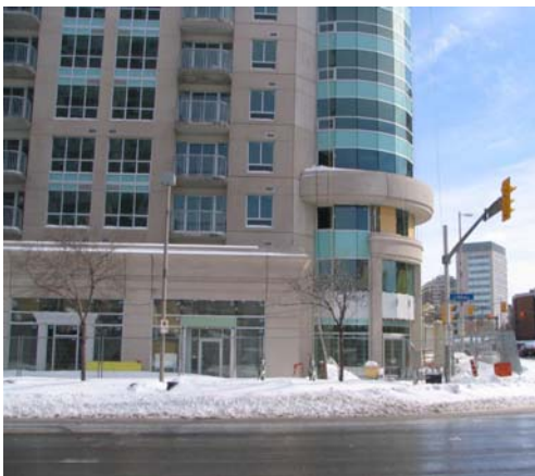
On Rideau Street, new retail space is being added at the podium level of two condominium projects, including Claridge Plaza (shown above).
