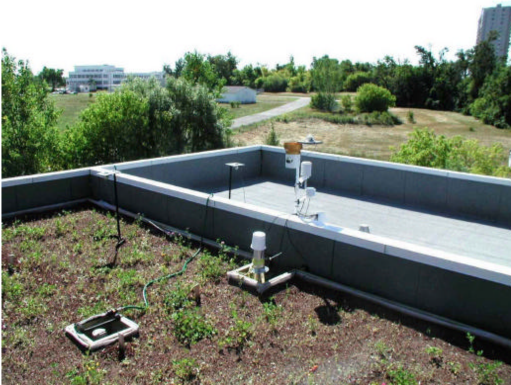
The Field Roofing Facility at the NRC campus in Ottawa. The median divider separates the Green Roof (left) and the Reference Roof (right). The weather station is located at the median divider.
